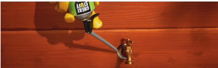
Water Faucet Penetration
